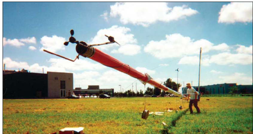
Installation of a 40m measurement mast
