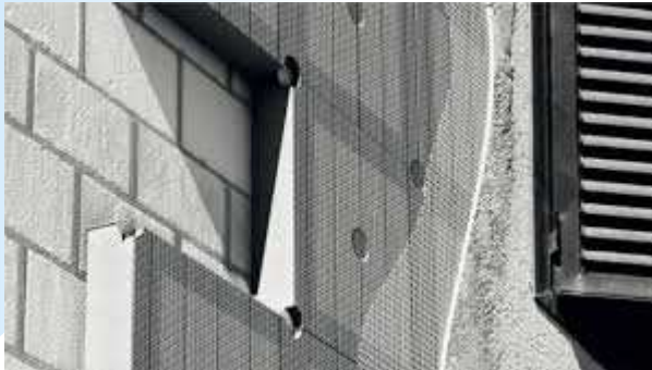
THERMAL COAT REALIZATION
