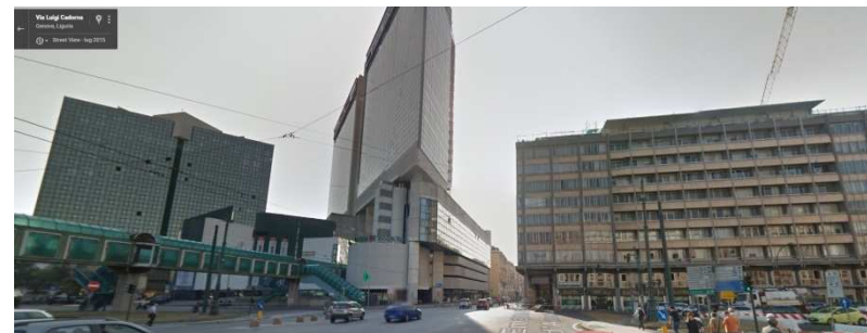
CONSTRUCTION OF YEARS '70 / '80
