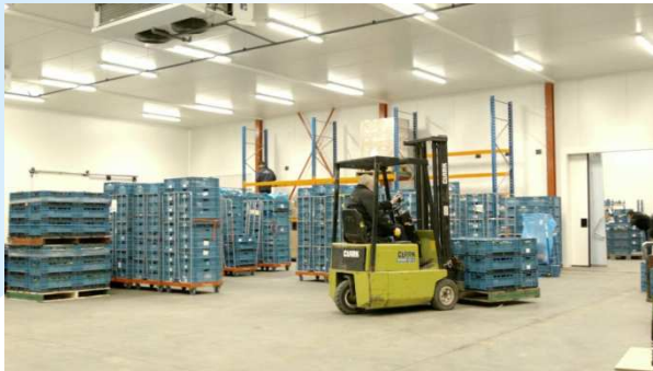
REPLACING A LED LIGHTING
