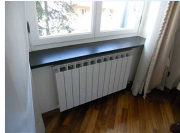
TERMINAL DELIVERY OF RADIANT ALUMINIUM TYPE
