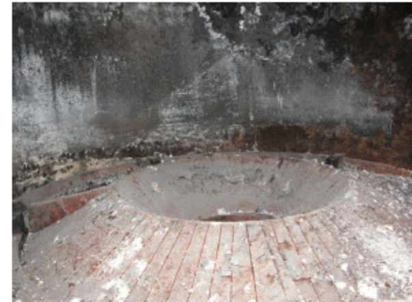
Furnace A: Underfed Stoker
