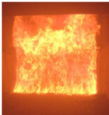
Furnace B: Moving Chain Grate
